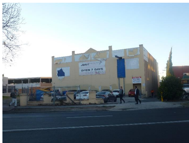
Figure 10: Existing development from the south east
