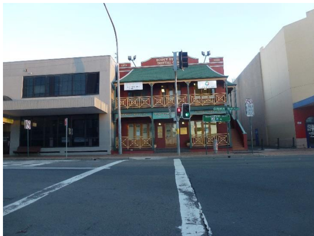
Figure 15: Two storey commercial building to the east of the George Street through site link
