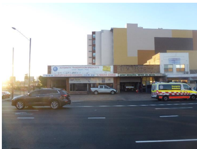
Figure 21: Rear party wall presented to the site
