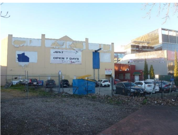
Figure 8: Rear car park of the commercial building as viewed from Terminus Street (south east)
